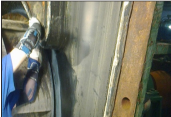
Existing rubber liners
